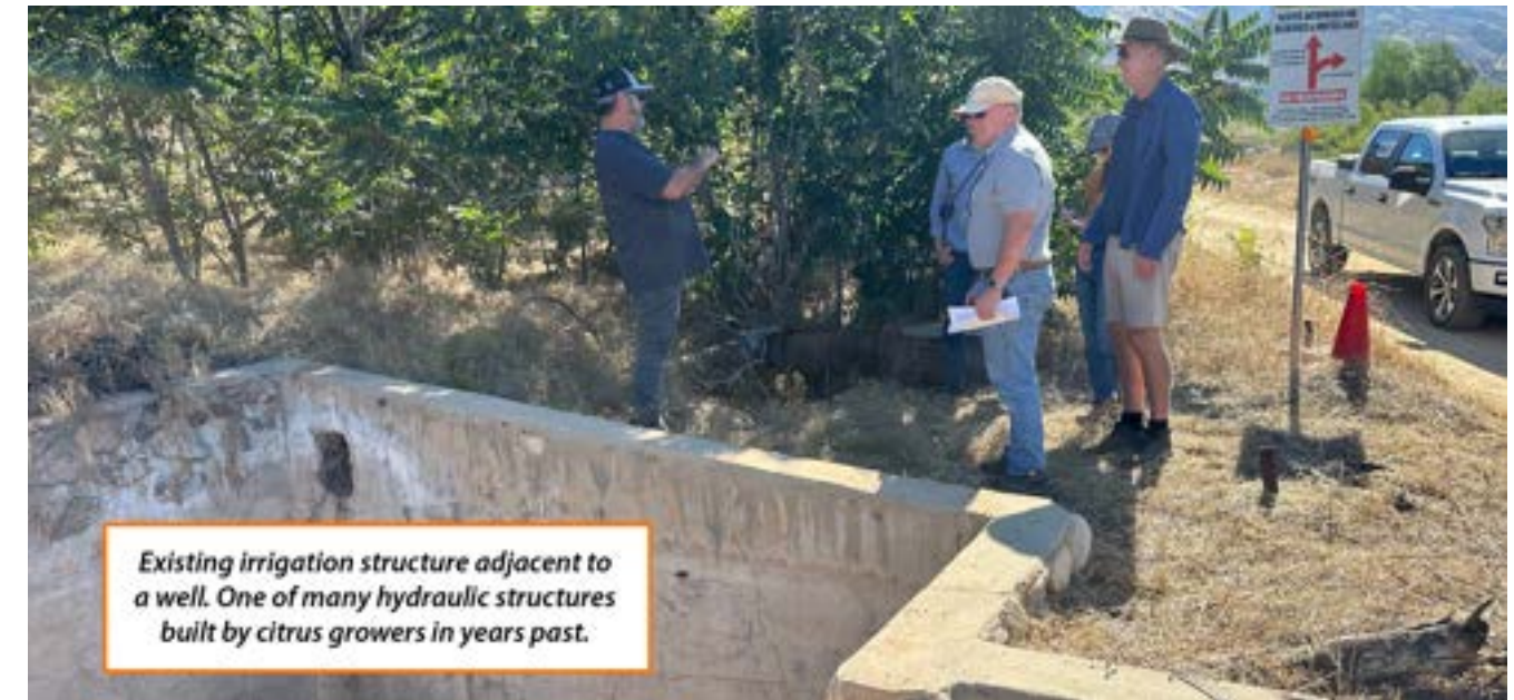
Figure 7-78 Existing agricultural well and structure
