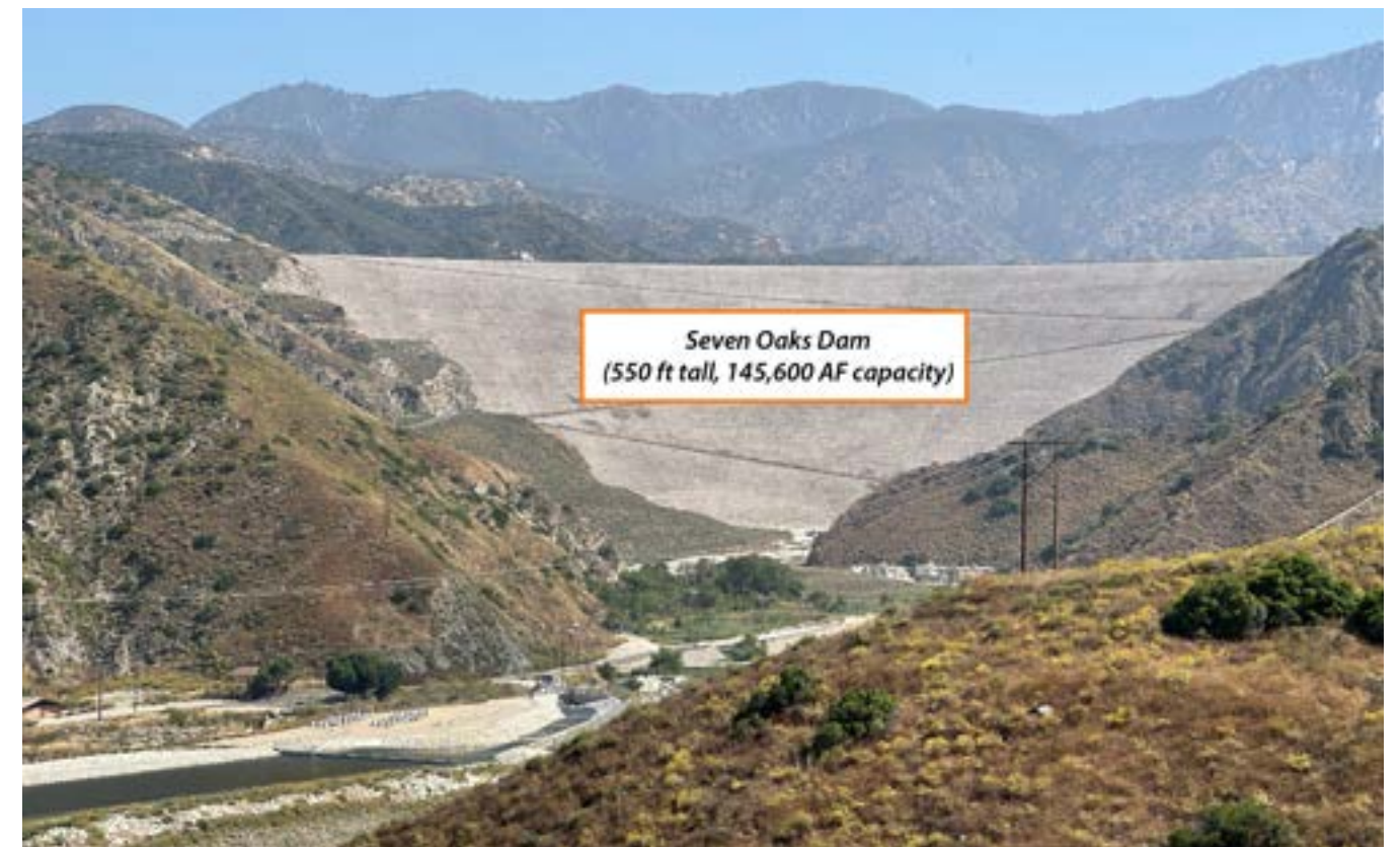
Figure 7-63 Seven Oaks Dam viewed from the south
