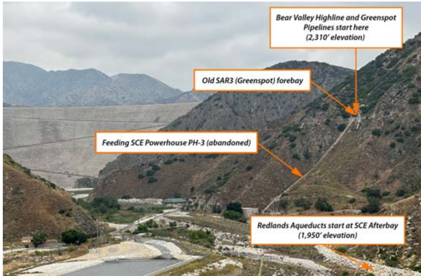
Figure 7-71 SCE Forebay Pipeline to Bear Valley Highline
