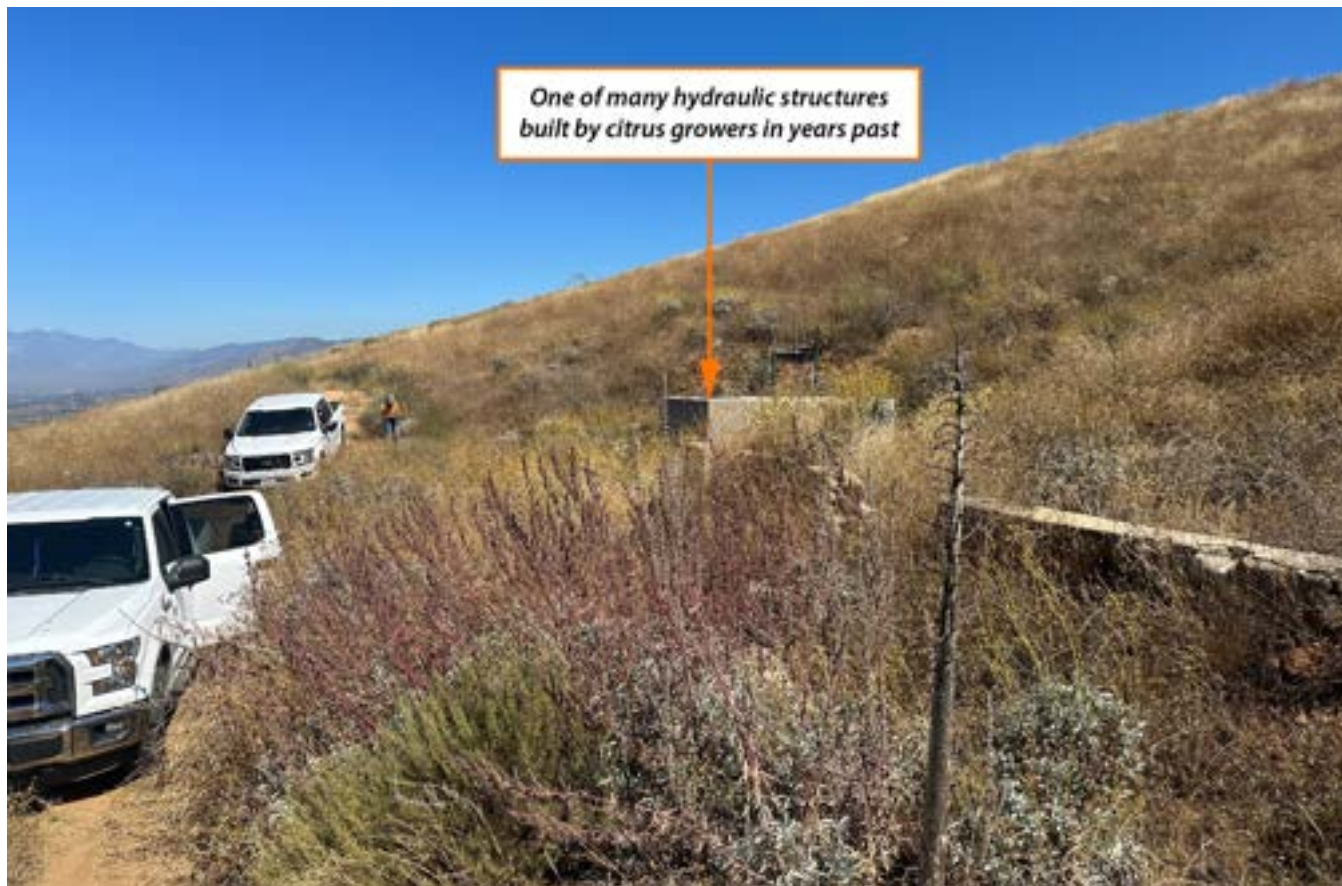
Figure 7-82 Bear Valley Highline Pipeline
