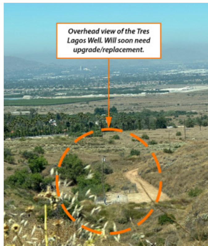
Figure 10-14 Tres Lagos Wells, access road, and power line
