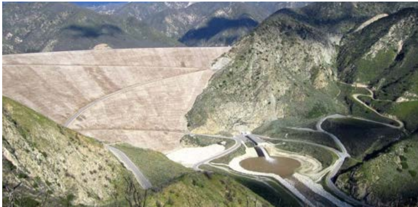
Figure 6-9 Seven Oaks Dam; Source Steve Schumaker, 2007
