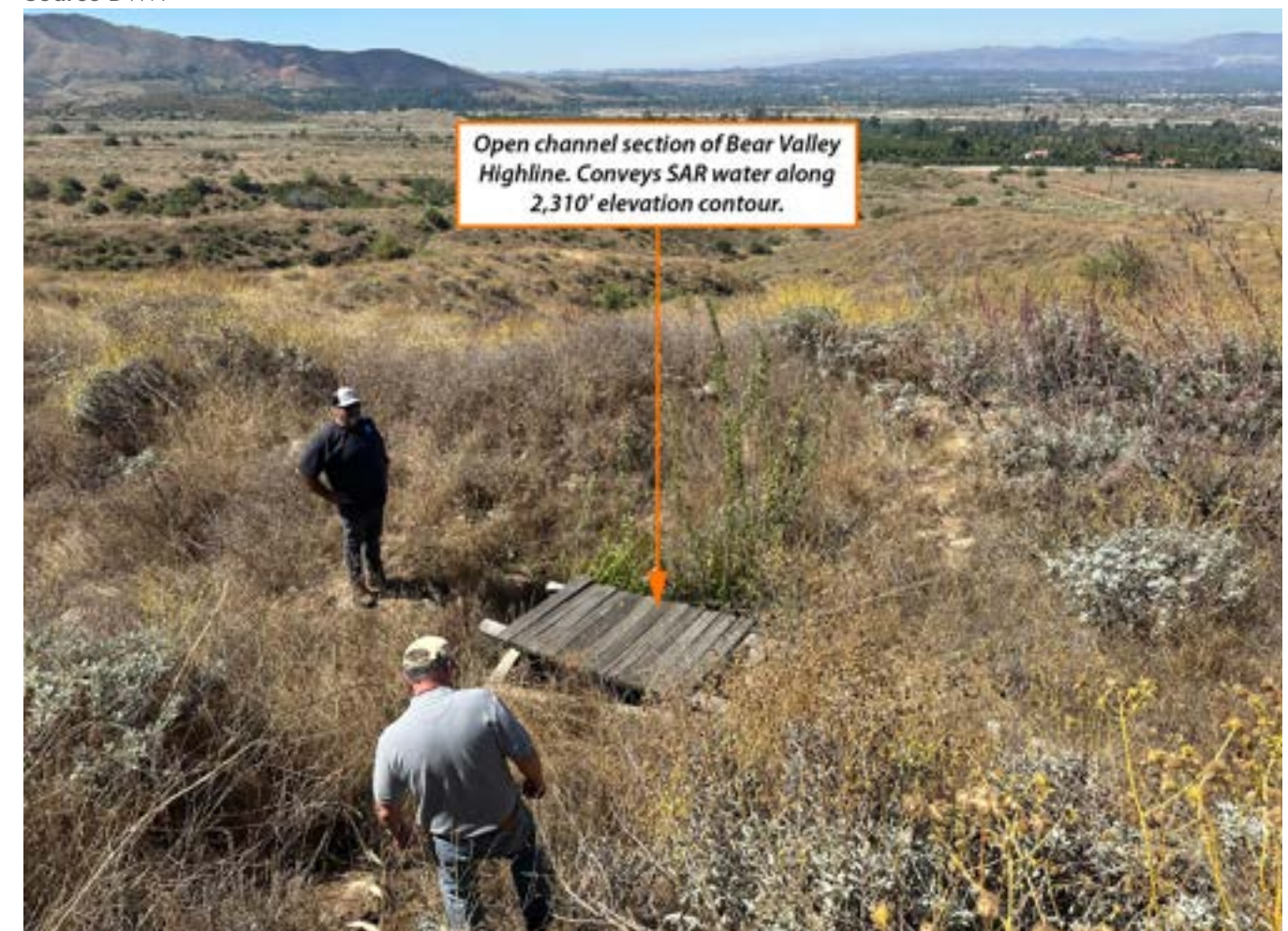
Figure 7-51 Bear Valley Highline Pipeline
