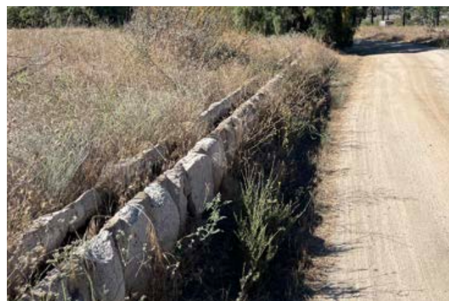
Figure 7-16 Irrigation canals created for the orchards
