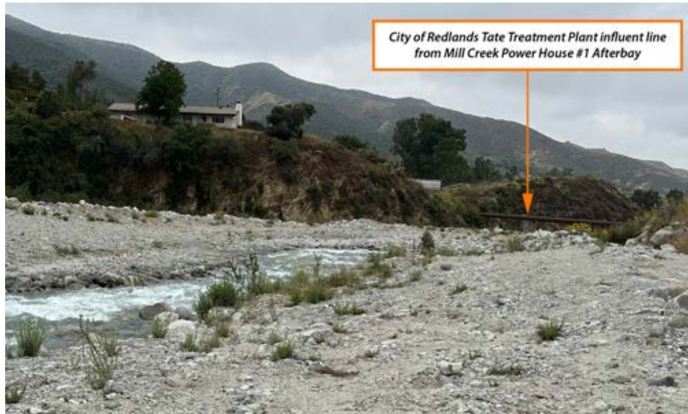
Figure 7-76 Mill Creek: View Looking Downstream from SCE Powerhouse #1
