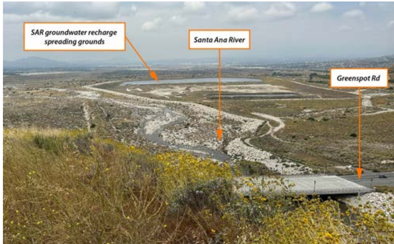
Figure 7-27 Santa Ana River at Greenspot Road Bridge: view of Santa Ana River Enhanced Recharge in the distance
