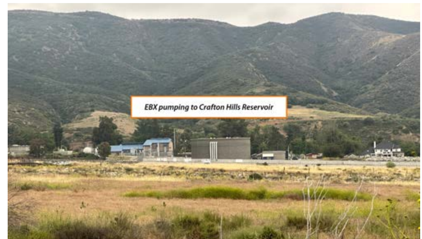
Figure 7-53 Tate & Crafton Pump Station on south side of Mill Creek
