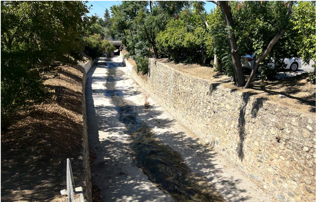
Mill Creek Zanja
