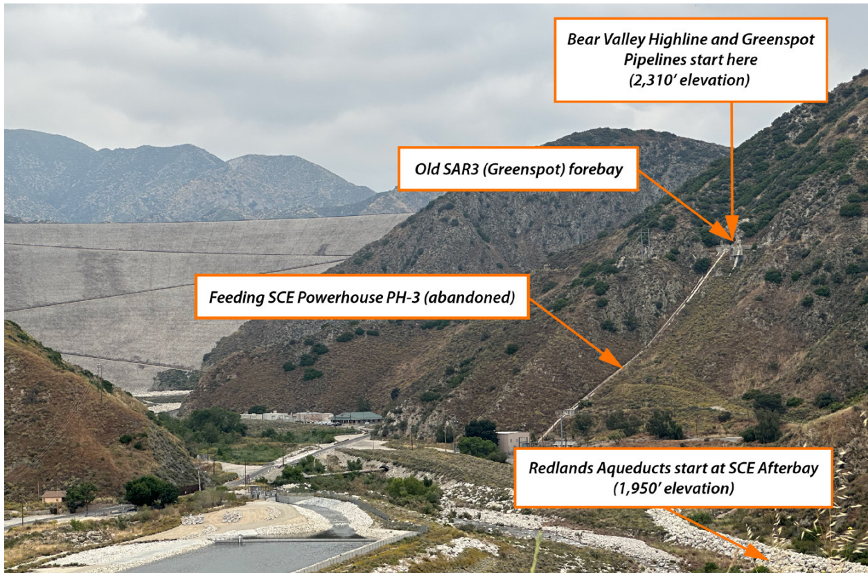
Figure 9. Powerhouse 3 Forebay Pipeline to Bear Valley High Line
